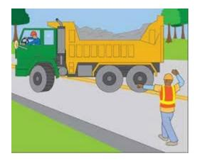
Many accidents involve the use of heavy equipment and machinery, and most of these accidents occur when a spotter is not used. Every worksite has its own specific hazards that present a great risk to equipment operators and ground workers.
